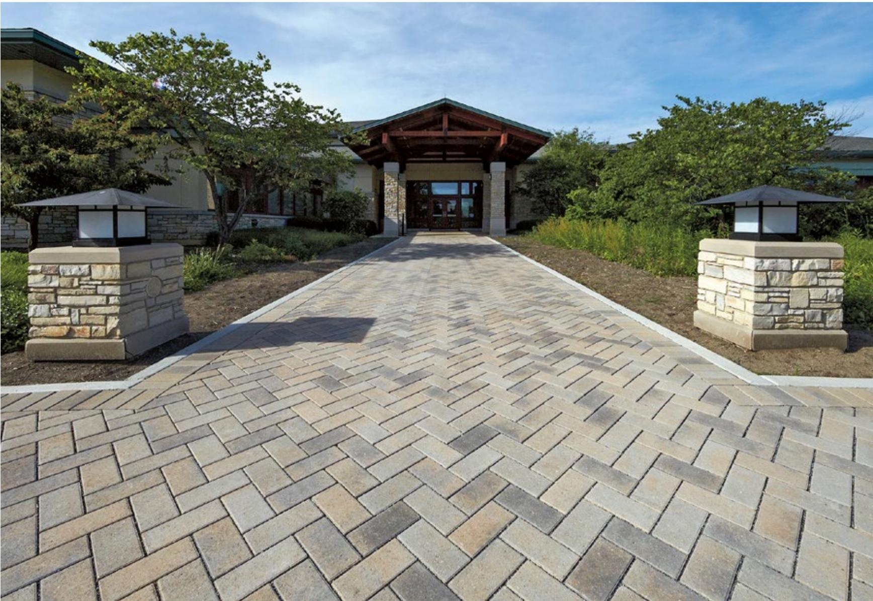
**USING PERMEABLE PAVING** for residential driveways and streetscapes not only allows builders to increase the size of the impermeable building footprint, but it also reduces the cost of stormwater management infrastructure.
