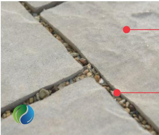
The pavers used in a permeable installation look very similar to traditional pavers, but are made with extra space between them so rainwater can flow back into the earth below, instead of running off the surface into storm sewers.
