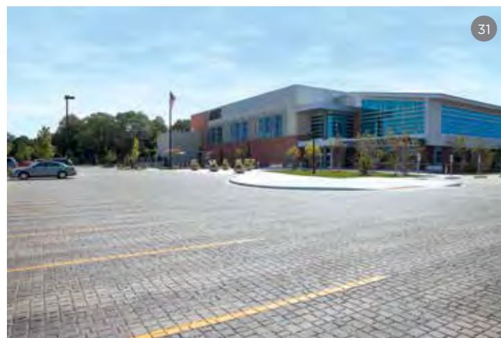
PROJECT: Athletic & Recreation Center. Woodridge, IL
