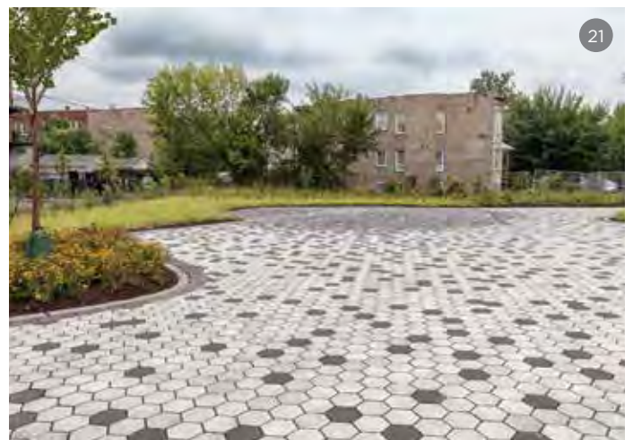
PROJECT: DPD Resilient Corridors Site 7. Chicago, IL
