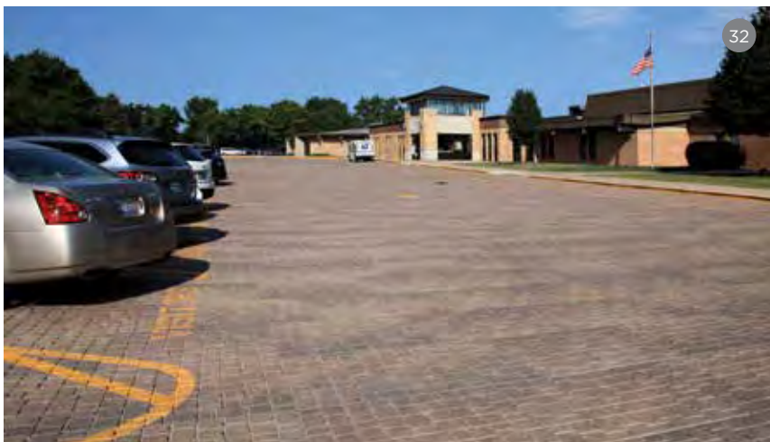
PROJECT: Jay Stream Middle School. Carol Stream, IL
