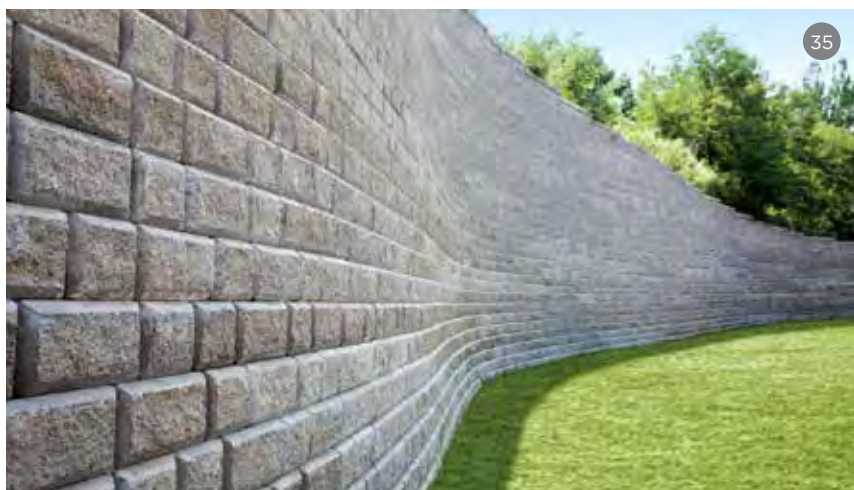
PROJECT: Victor Crossing. Victor, NY
