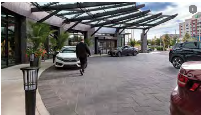
PROJECT: Residence Inn by Marriott. Columbus, OH
